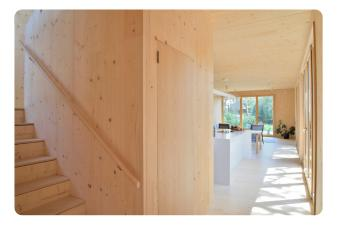
Tilly 3-Ply Spruce 'CLT' sheets are the standard LAROS wall and ceiling linings. Wall and roof panels are always constructed with a 3-ply lining that can then be covered with the desired architectural finish. Floor panels can be fitted with commonly available structural floor and ceiling sheets on request.
