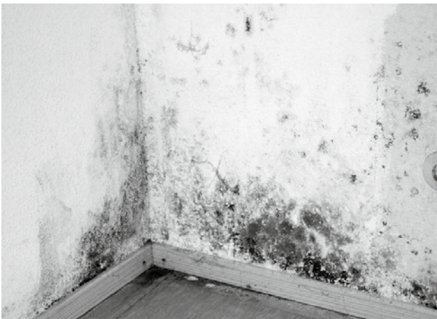
Examples of physical manifestation of fungus attack at thermal bridge areas.
