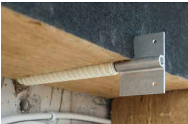
Rainscreen cladding facade attached with Schöck Isolink® type TA-S: Multi-purpose hall, Volkertshausen Germany. ©Schöck Bauteile GmbH
