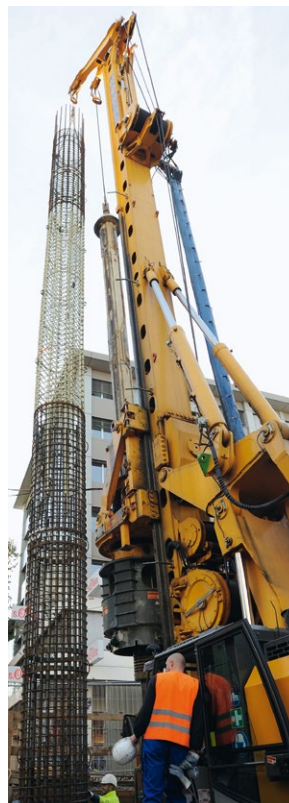
Light rail tunnel Karlsruhe, Germany
