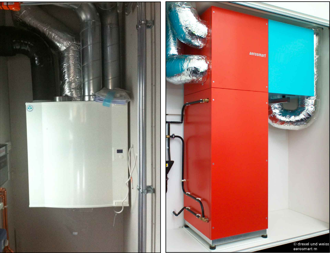
ERV UNIT INSTALLATION EXAMPLES
