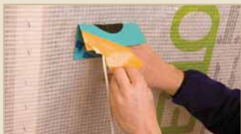
Fig. 90. ROFLEX pipe grommet fixed with TESCON VANA
