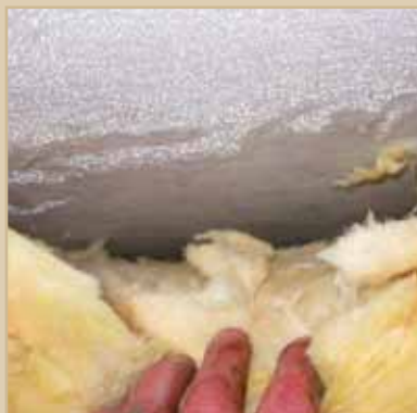
Microporous membrane – Passive diffusion transport: Wet – condensation
