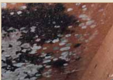
Fig. 3. Mould in the building structure
