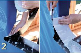
Cut TESCON EXTOSEAL to appropriate length (sill length plus required jamb height on either side).
