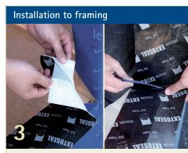
Remove first release foil to allow for application onto sill and jamb framing. Start installing the Sill Tape from the first preinstallation measurement of the first jamb. Follow the sill and up the second jamb. Ensure you apply the Sill Tape tightly into the corner and smoothly along the sill frame using the pro clima PRESSFIX.
