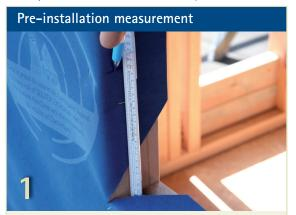
Measure vertically up the jamb from the internal corner of the sill. Minimum 100 mm allowing for 50 mm cover onto the wall underlay.
