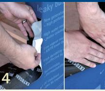
Remove second release foil to allow for application onto weathertightness layer. Fold and stretch to the face of the weathertightness layer. Ensure you apply the Sill Tape smoothly using the pro clima PRESSFIX.
