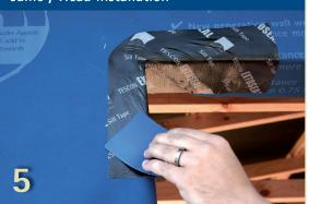
Measure vertically down the jamb and horizontally across the head trimmer from the internal corner. Minimum 100 mm allowing for 50 mm cover onto the weathertightness layer. Repeat installation to jamb and head trimmer as per steps 3 and 4. If you have any questions, please call our technical hotline **0800 PRO CLIMA.**
