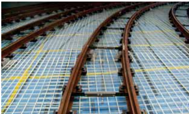
Floor slab railway depot Basel, Switzerland
