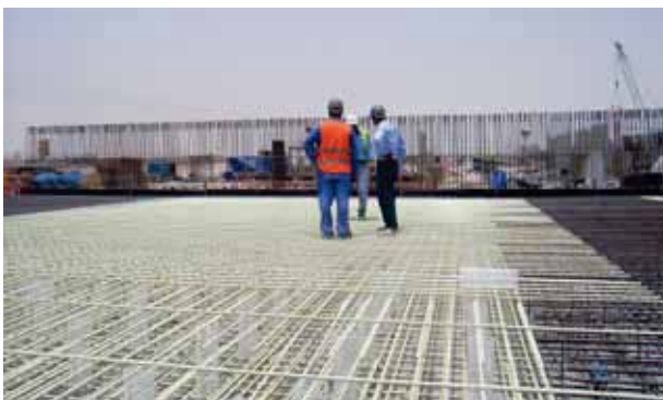
Floor slab in rectifier area Qatar Aluminum, Qatar
