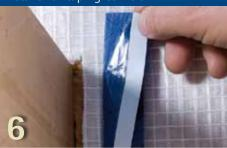
Seal corners using pro clima TESCON PROFIL tape. Remove one strip of the split release paper and press down the first piece. Then remove the second strip of the release paper and press down the second piece.
