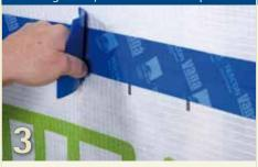
The TESCON VANA tape should be applied centrally and pressed down firmly using the pro clima PRESSFIX.
