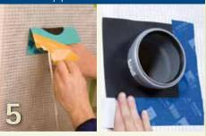
Seal all round penetrations with KAFLEX or ROFLEX grommets.
