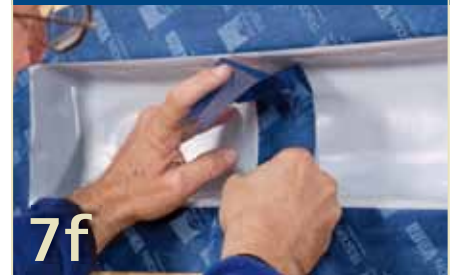
Enlarging: Taping over the overlaps
