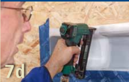
Enlarging: Fixing the overlap
