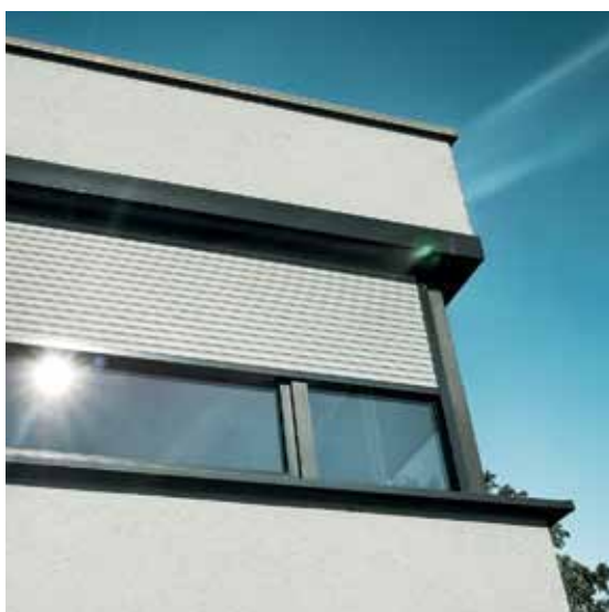
PENTO head box installed flush with the façade (requires a certain wall thickness)
