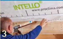
The liquid adhesive ORCON is applied to join the INTELLO® membrane to concrete or wooden frames. Do not press the adhesive completely flat.
