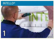
The INTELLO® airtightness membrane is laid on the interior, over the insulation. Bonding with adhesive tapes should be on the smooth printed side. Staples should be 10 mm wide and 8 mm long and set at a max distance of 100 mm -150 mm.
