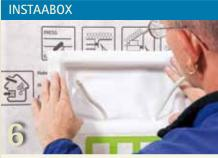
The airtightness box for power points and light switches is cut and fitted into the INTELLO® layer and then sealed by using TESCON VANA to create a seamless airtightness system.
