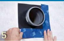
ROFLEX pipe grommets are affixed using TESCON VANA. Press firmly to secure the adhesive tape.
