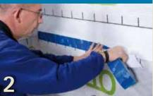
Seal the membranes at overlaps without strain or loading, using TESCON VANA adhesive tape. The tape should be applied centrally and pressed down firmly using, for example, pro clima PRESSFIX.
