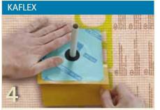
If pipes or cables penetrate the airtightness layer, they too must be securely sealed. KAFLEX cable grommets are self-adhesive. Remove the release paper, push over the cable and stick on.
